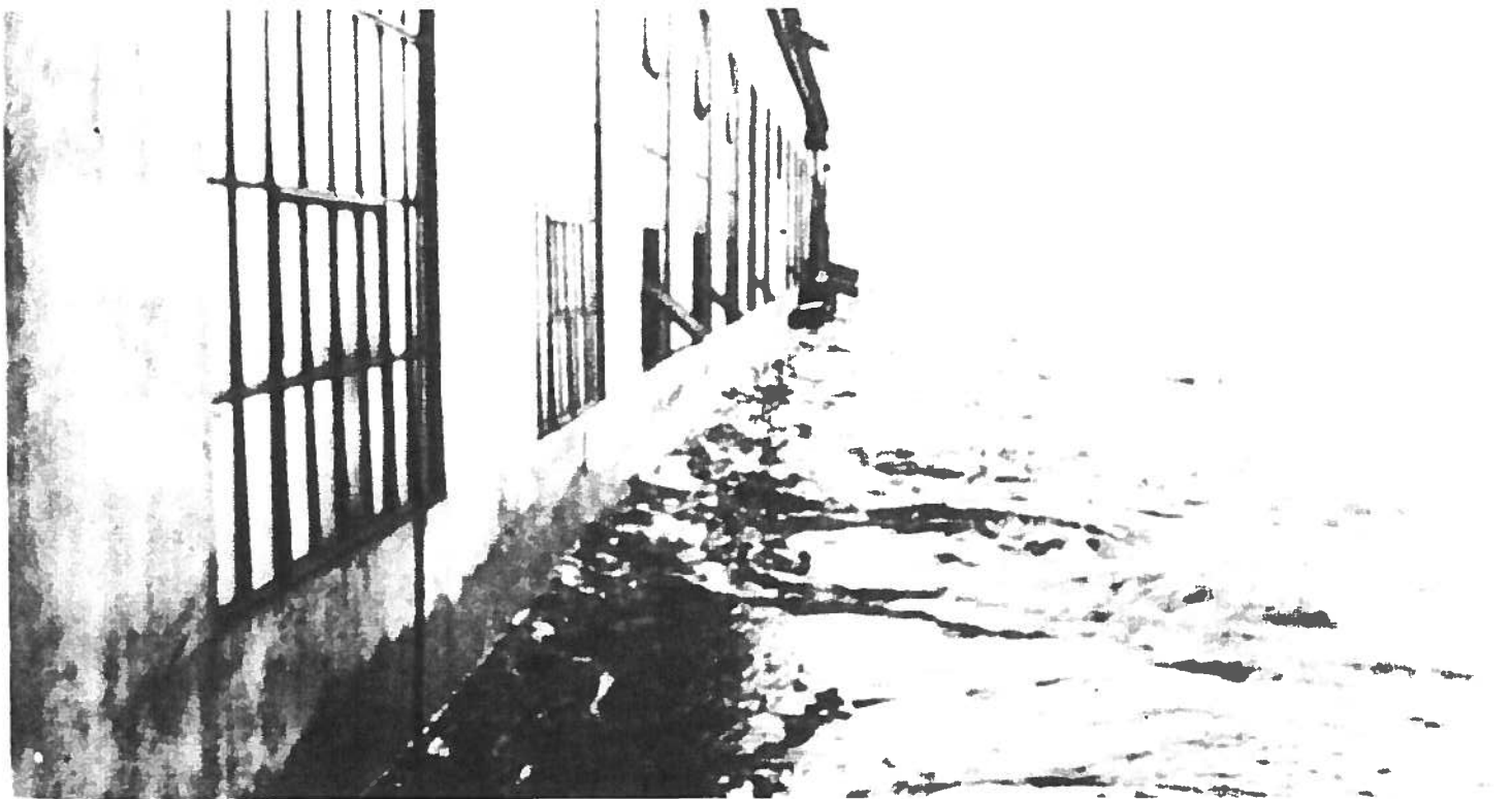
High water in Forebay at Veazie Station, showing outside wall of generator room. Platform which runs entire length of station used for track for rack rake under water.
